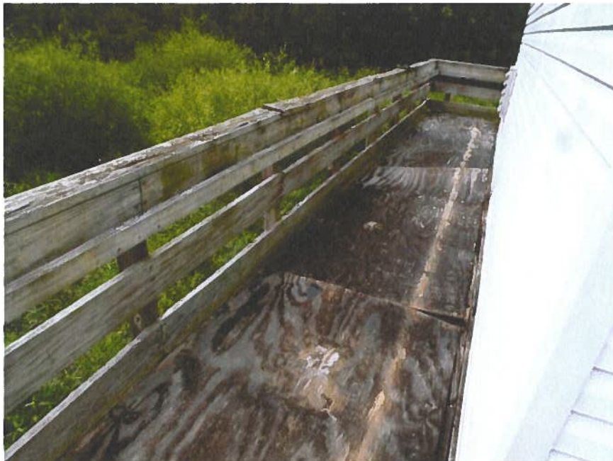
Photograph P – Pier/Dock Failing Boards
