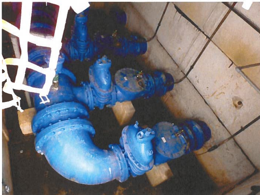
Photograph T –Transfer Pump Station Valve Vault
