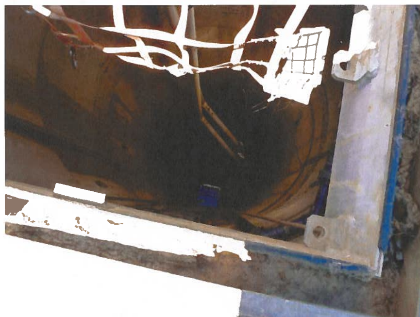
Photograph DD- NPDES Compliance Chemical Injection Vault
