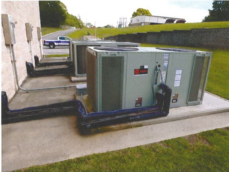
Photograph G – New Electrical Room HVAC Units
