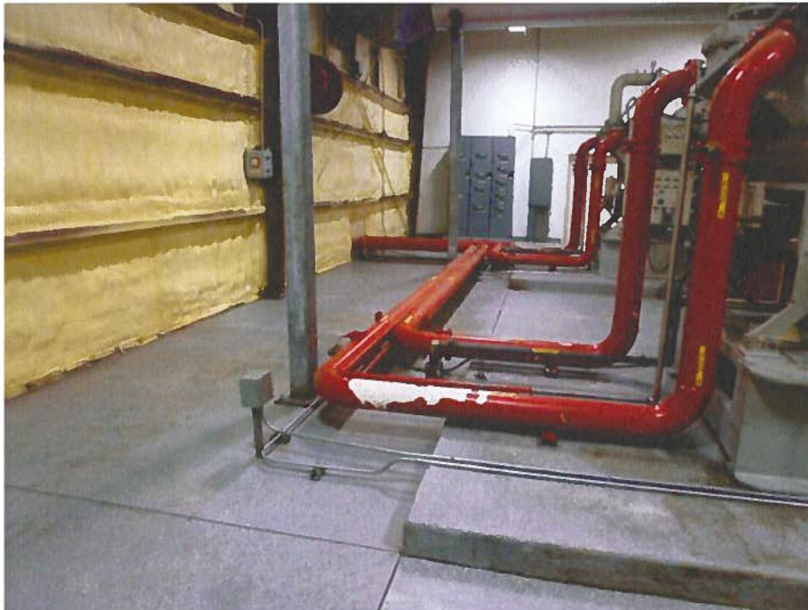
Photograph R – Generator Coolant Piping
