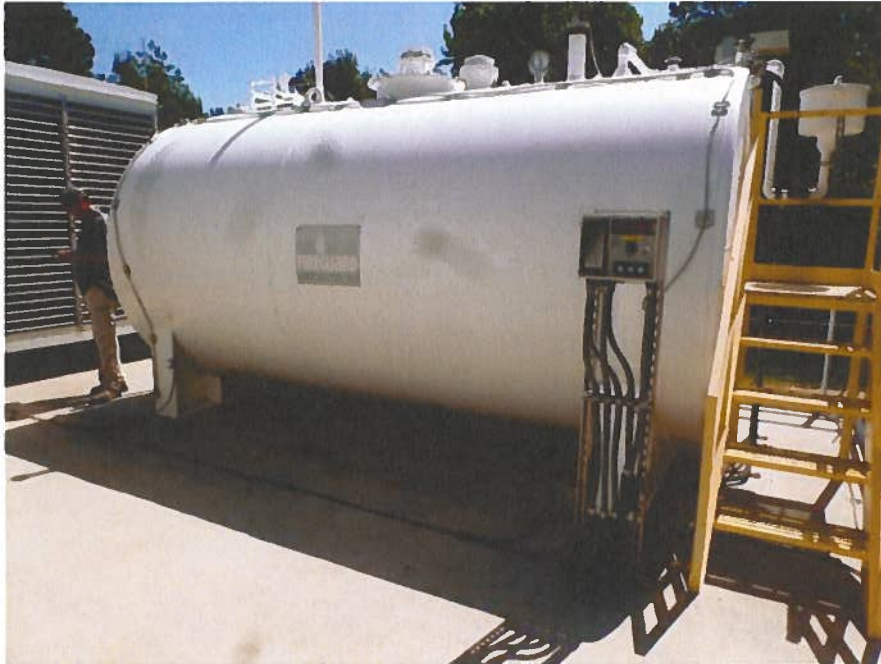
Photograph G – Raw Water Pump Station Generator Fuel Tank
