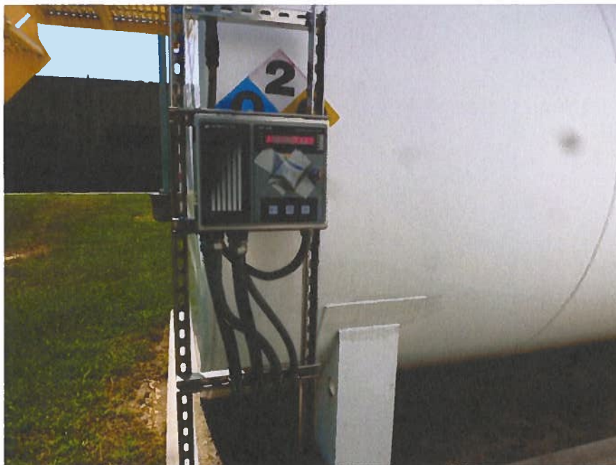
Photograph BB- Facility Generator Diesel Tank Leak/Level Panel
