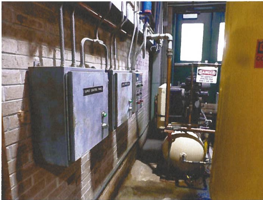
Photograph L- Surge Tank Controls
