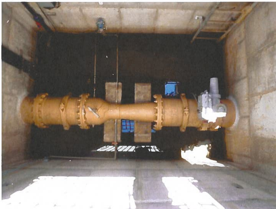
Photograph L – Influent Flow Meter Vault
