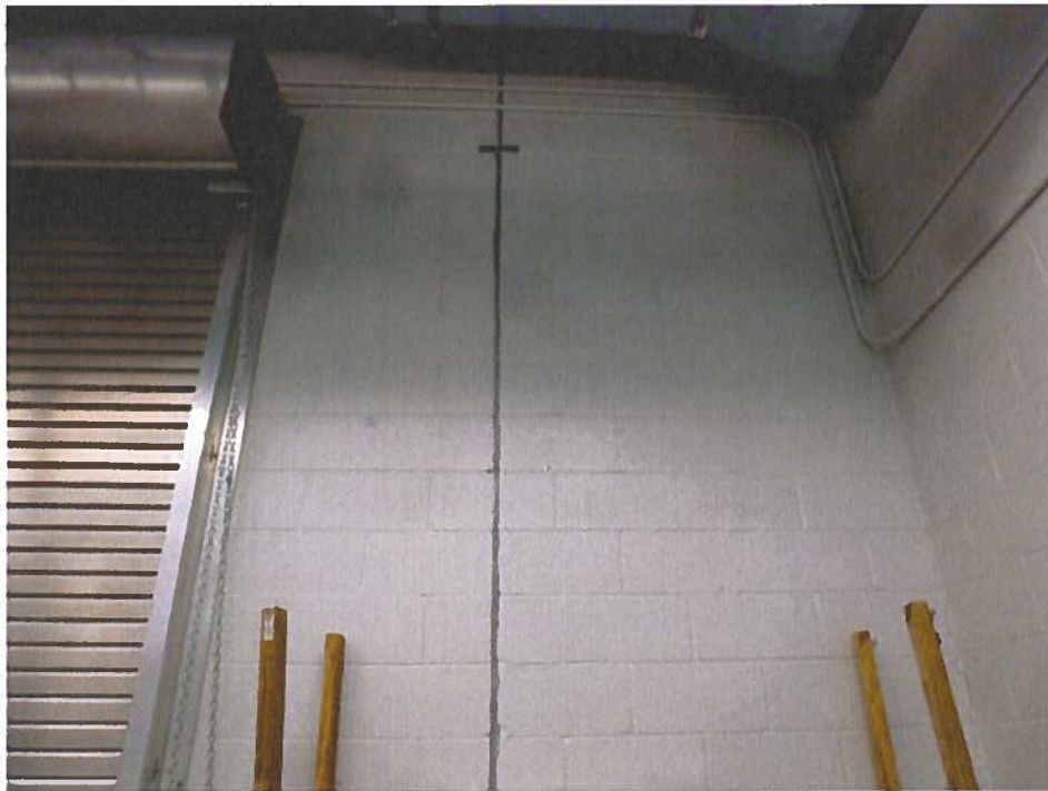
Photograph F – Masonry Control Joint in Electrical Room
