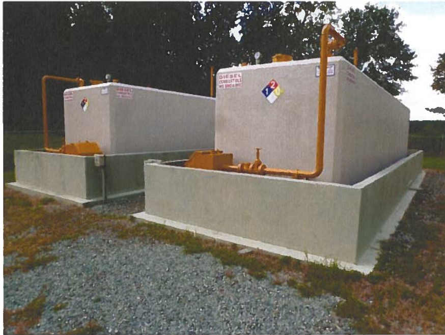
Photograph I – Generator Fuel Storage Tanks
