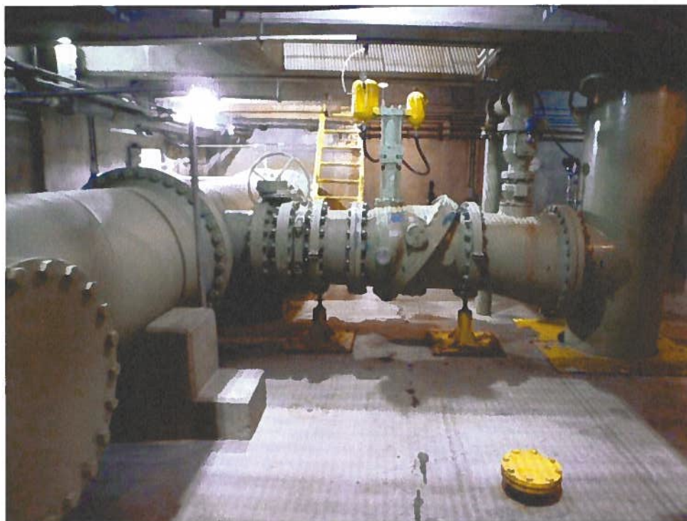
Photograph B – Check Valve on Pump #1 No Longer Leaking
