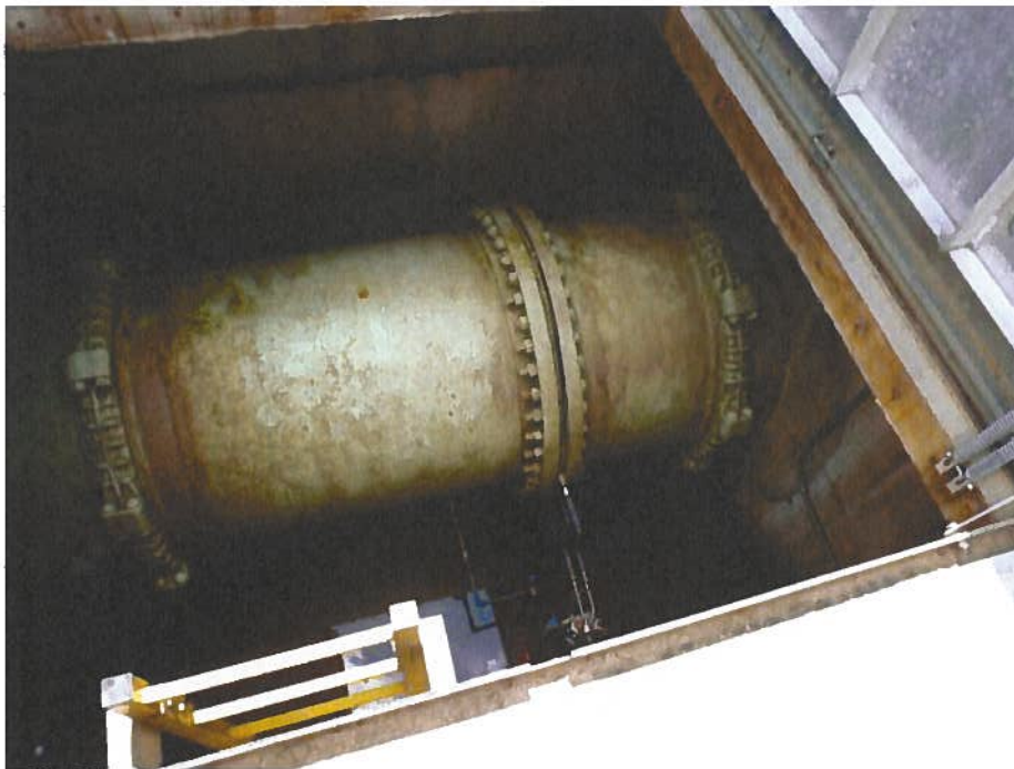
Photograph H –Effluent Pump Station Flow Meter
