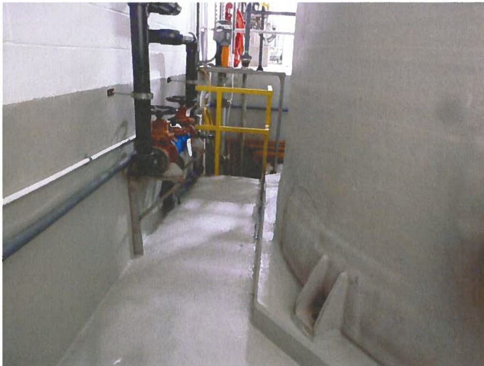
Photograph Z- Chemical Building Chemical Carrier Water RPZ
