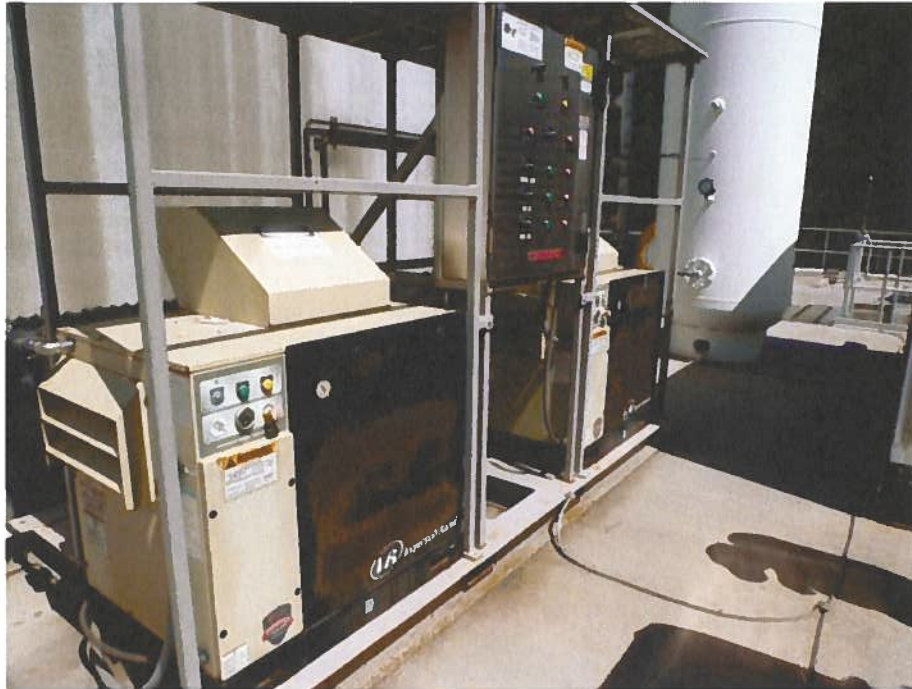
Photograph K -Raw Water Pump Station Backwash Compressor
