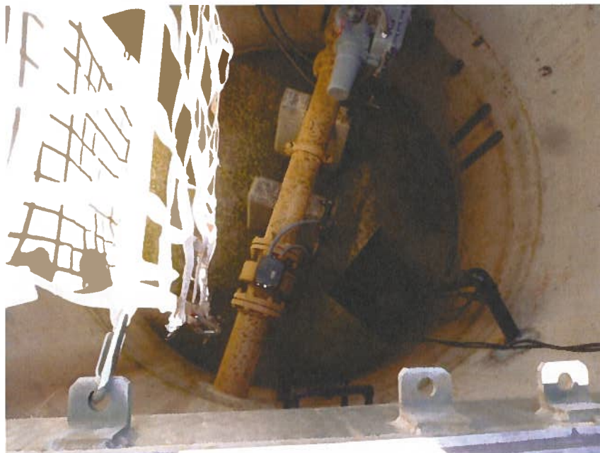
Photograph CC- NPDES Compliance Meter Vault
