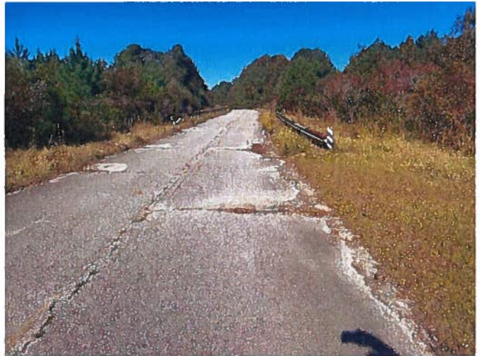
Interior Access Road
