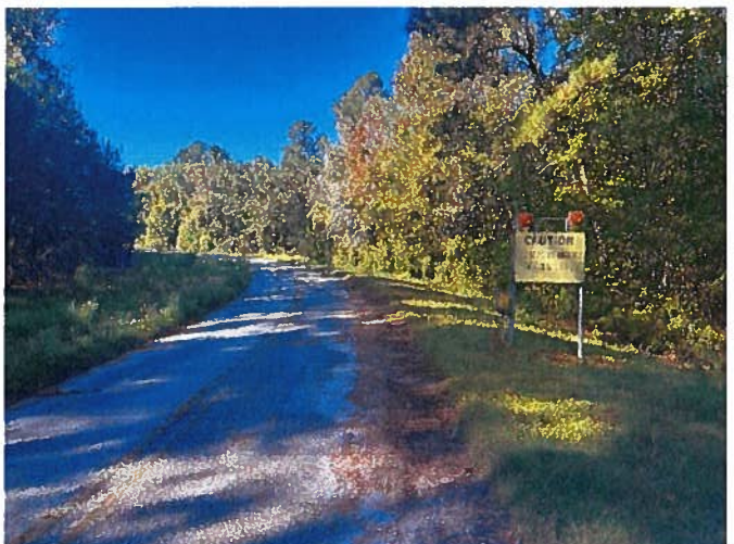
Interior Access Road
