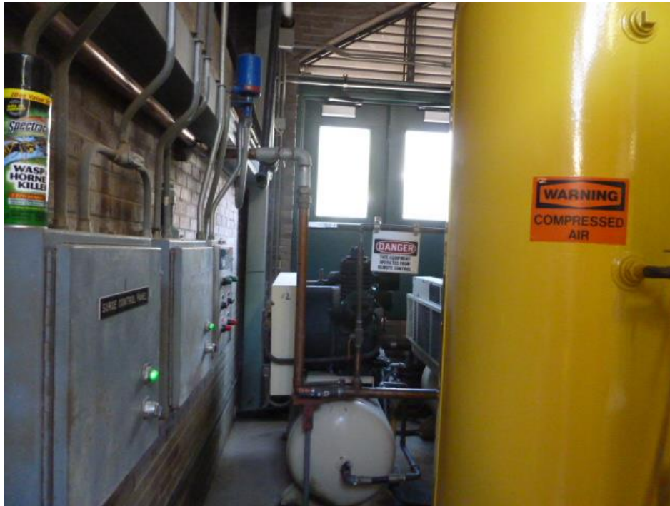
Photograph P – Surge Tank Drain Piping
