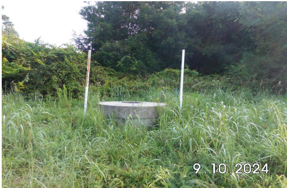
Photograph BB – Orange Painted Structure Marker Deterioration
