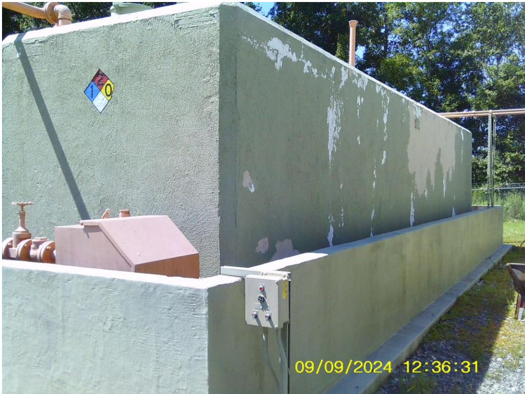
Photograph K – Diesel Storage Tank Coating Repairs
