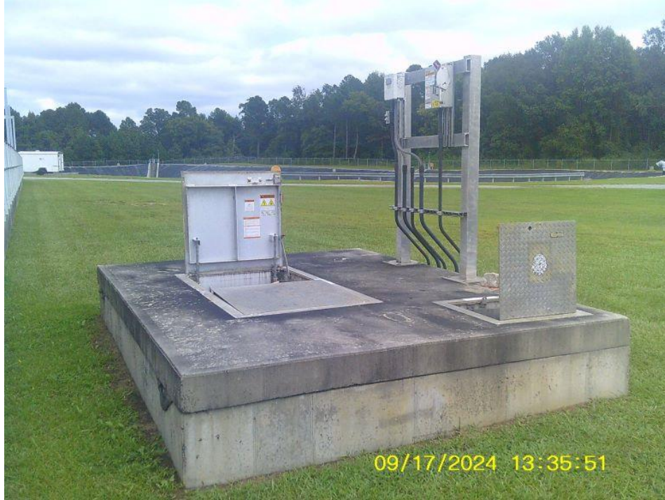
Photograph M – Influent Flow Meter Vault
