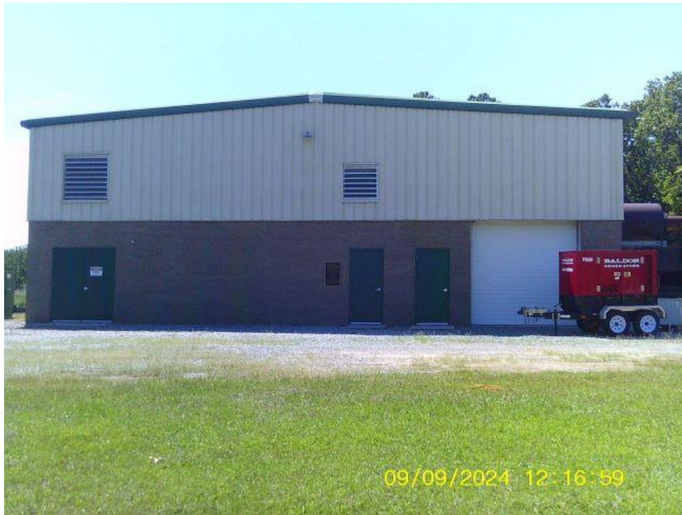
Photograph U – Generator Building Doors Replaced
