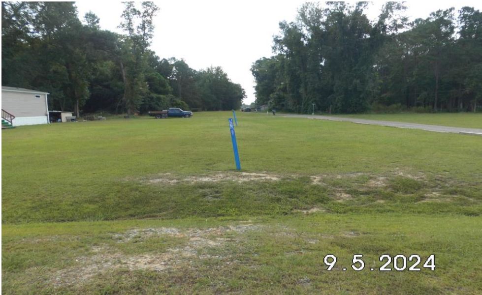
Photograph CC – New Blue Marker Post from 54" RWM project.
