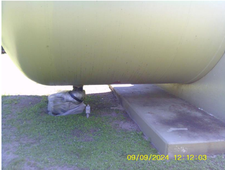
Photograph P – Surge Tank Drain Piping
