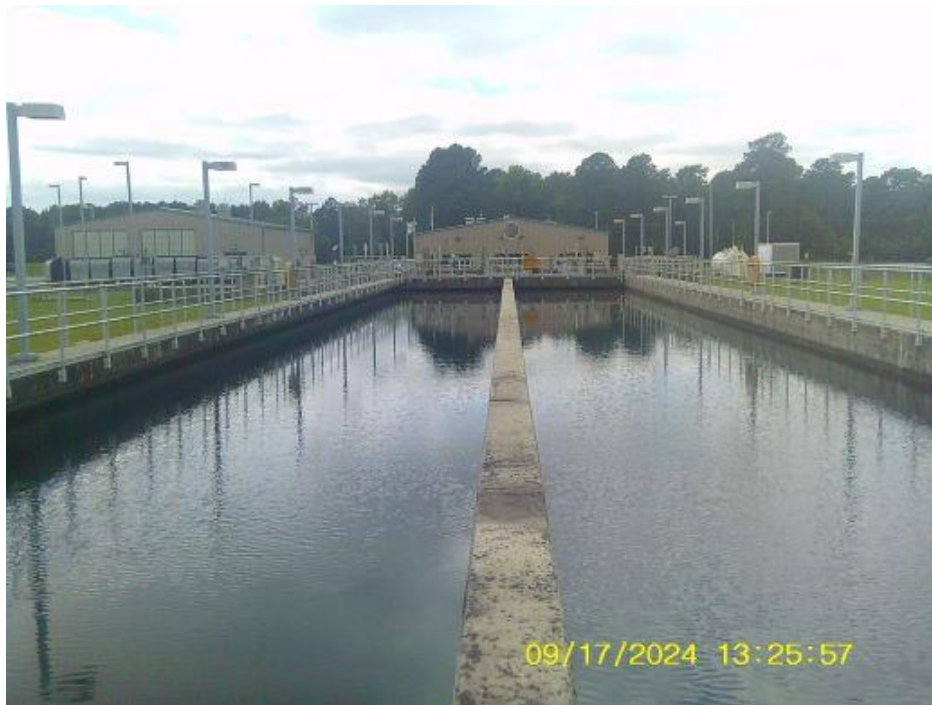
Photograph O – Sedimentation Basins
