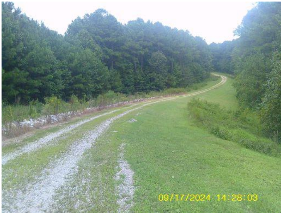
Photograph J – Access Road to Pump Station
