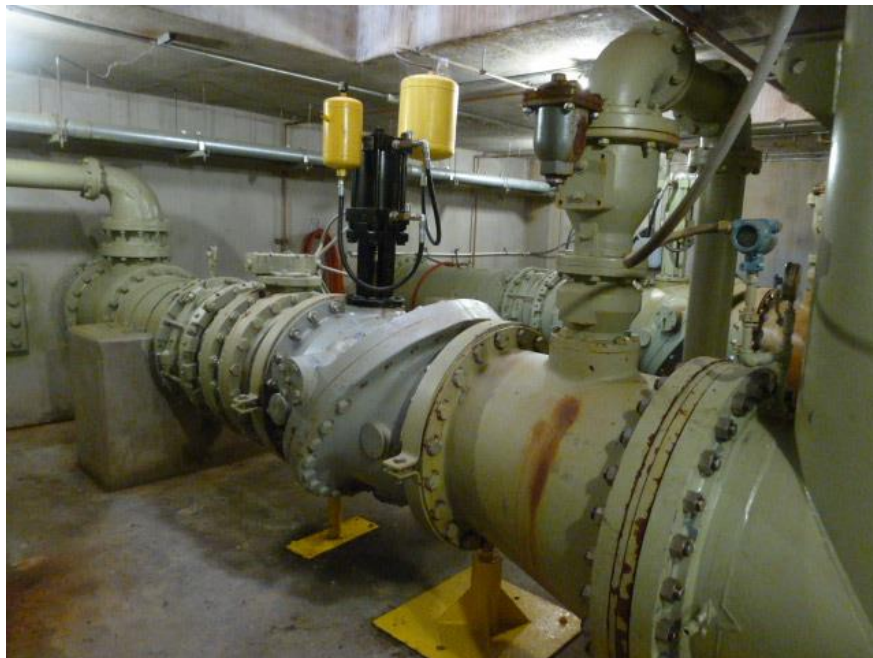
Photograph C – Failed Check Valve on Pump 5
