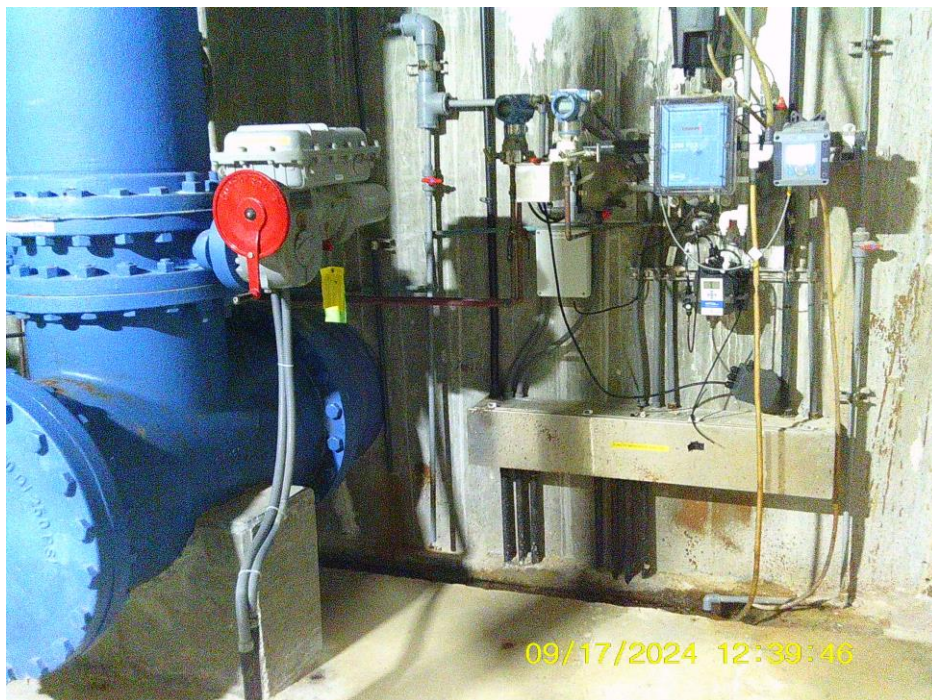
Photograph P – Filter Gallery Walls
