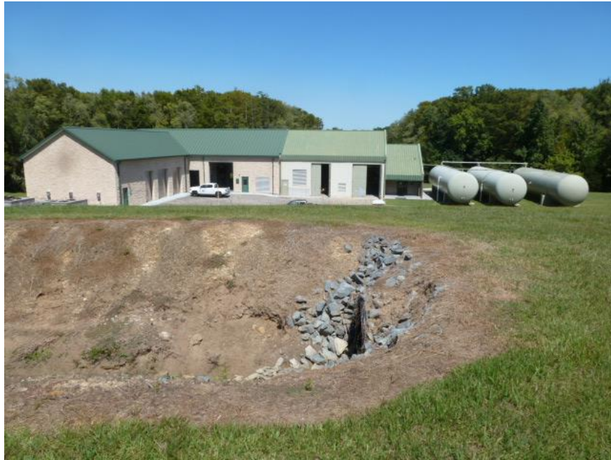
Photograph N- Ditch Access Walkway
