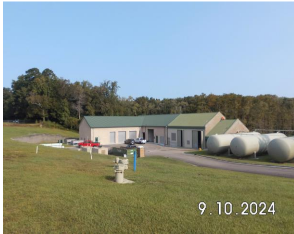
Kings Bluff Raw Water Pump Station
