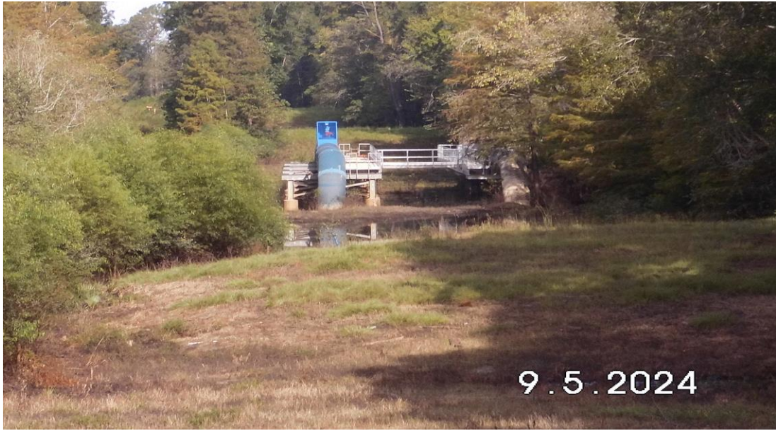
Photograph II- Walkway Access across Livingston Creek on Existing 48" PCCP pipe
