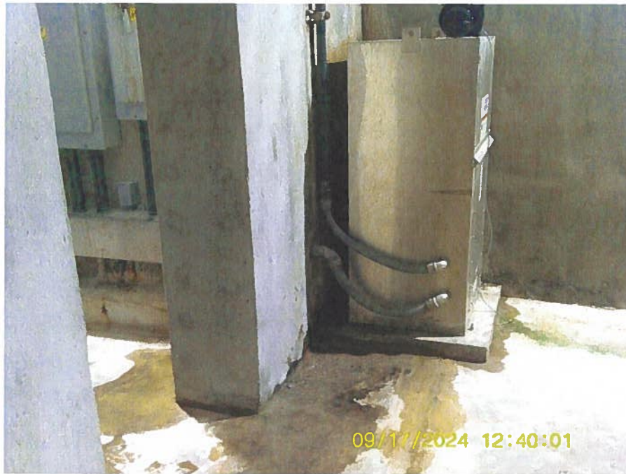
Photograph Q – Filter Gallery Wall Leaks
