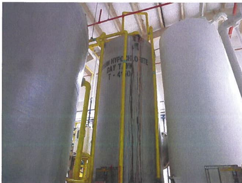
Photograph Z- Chemical Building Chlorine Tank Leak
