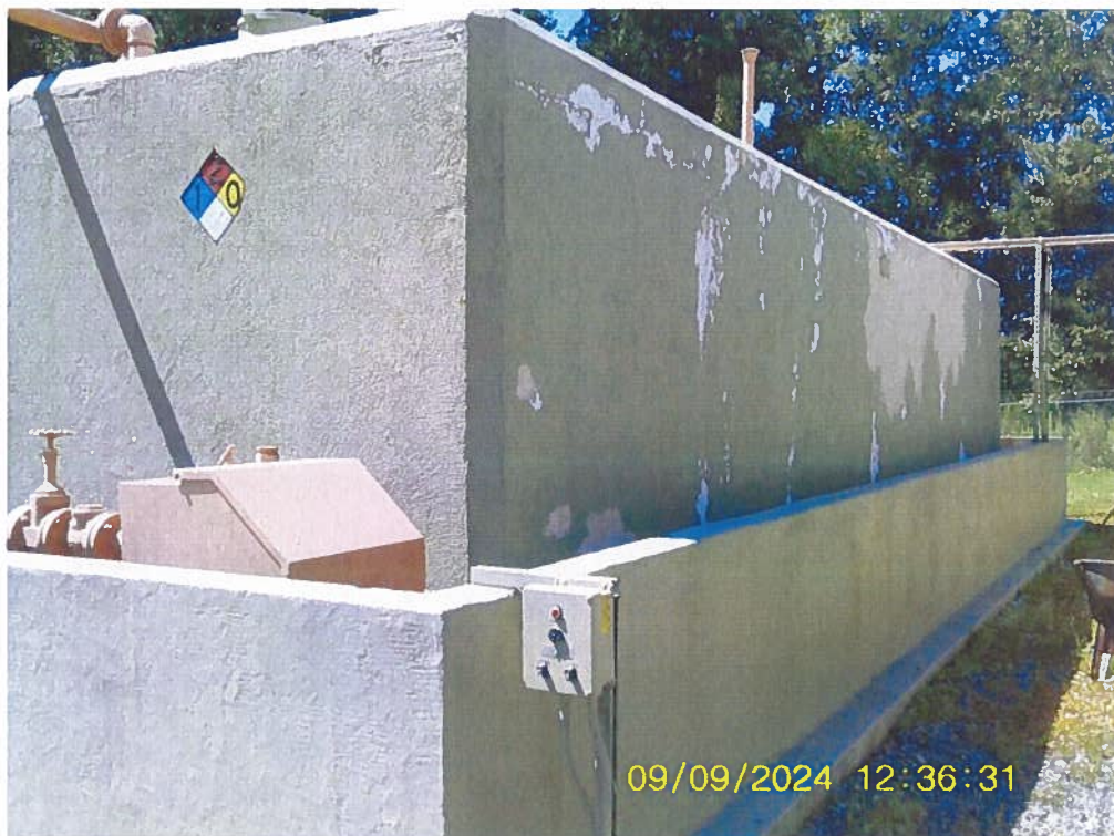
Photograph K –Diesel Storage Tank Coating Repairs
