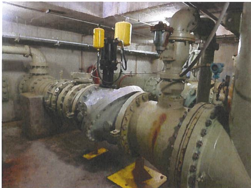
Photograph C – Failed Check Valve on Pump 5
