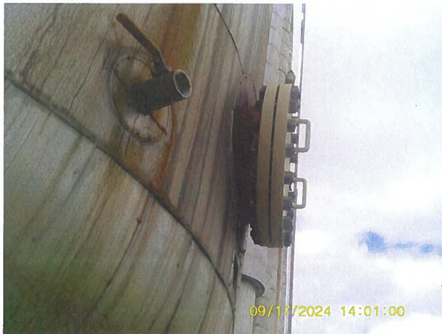
Photograph X- GAC Filter Manway Corrosion
