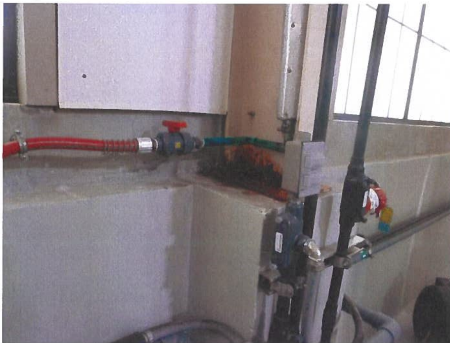
Photograph Y- Chemical Building Interior Piping Leak
