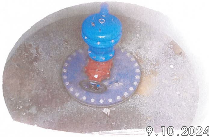
Photograph DD – Old ARV on 48" RWM and New ARV on 54" RWM
