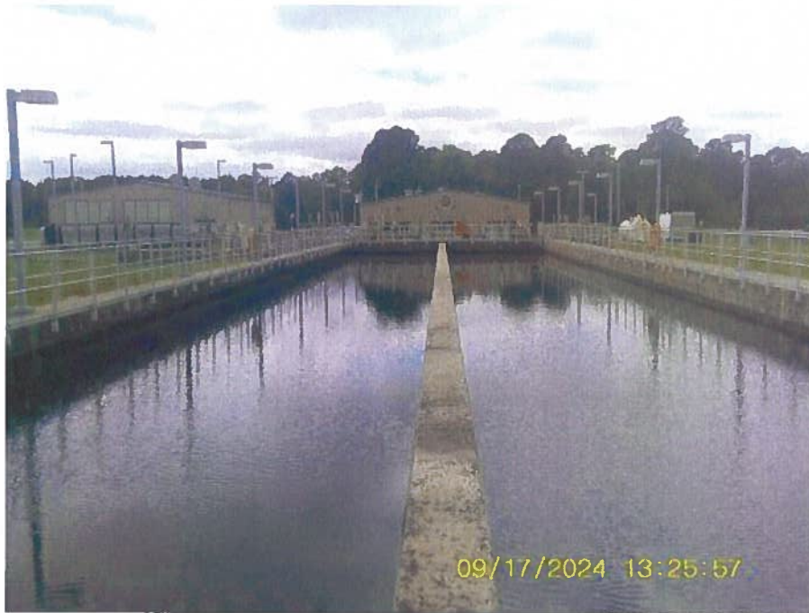
Photograph O – Sedimentation Basins
