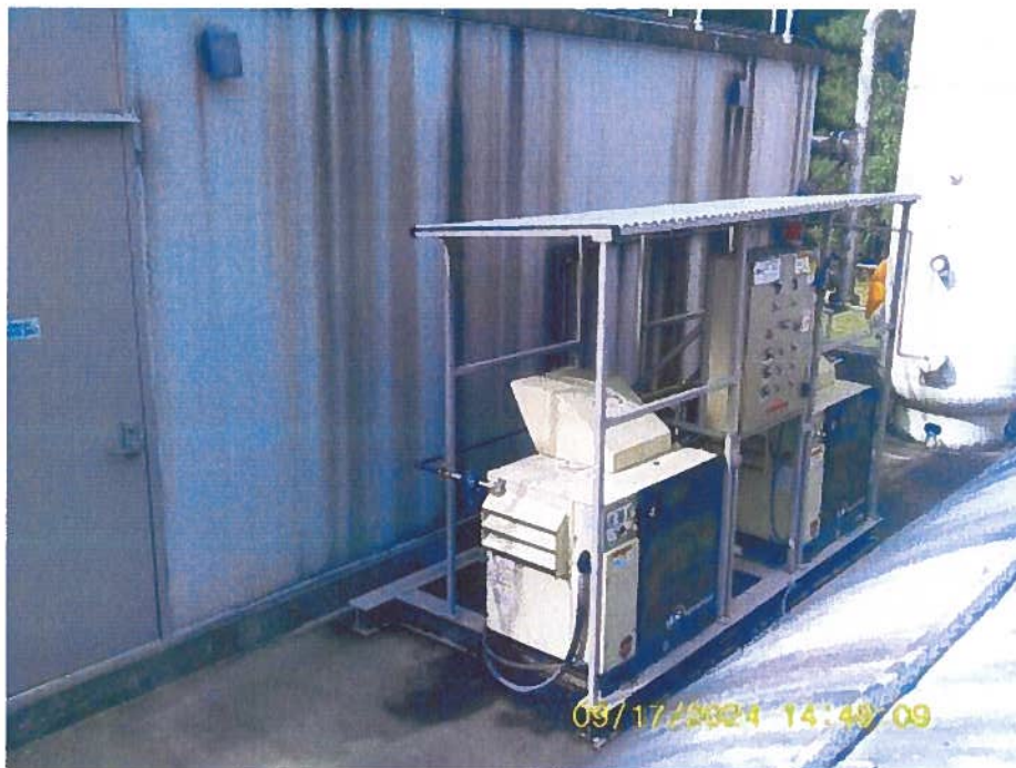
Photograph L – Air Backwash Compressor
