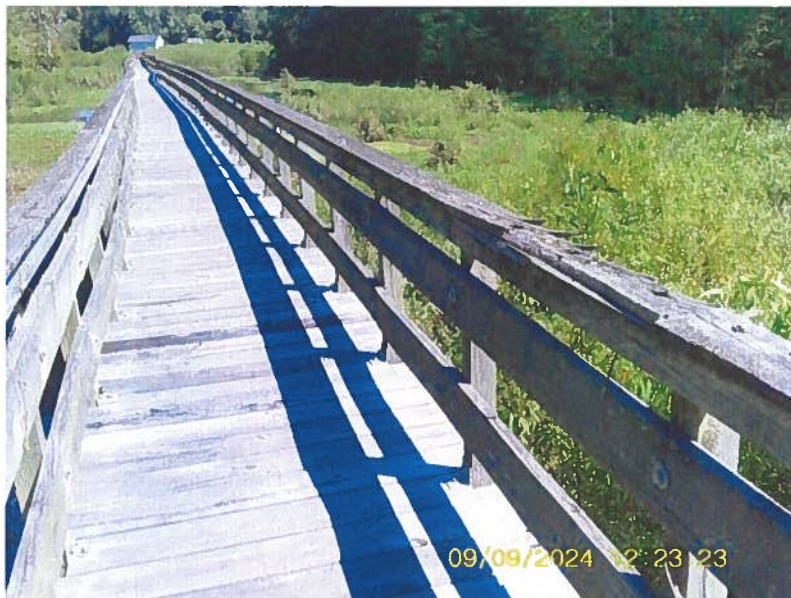
Photograph T – Pier Rotten Boards
