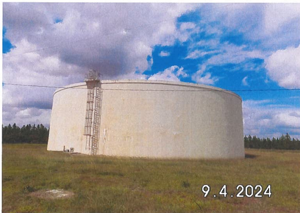
Photograph JJ- 3 Million Gallon Ground Storage Tank
