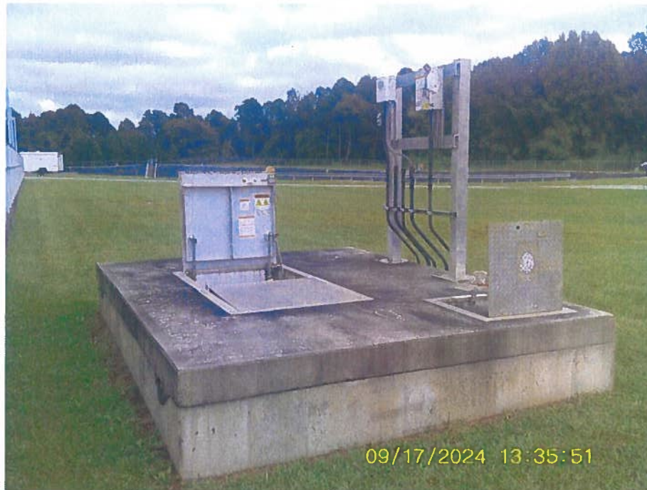
Photograph M – Influent Flow Meter Vault
