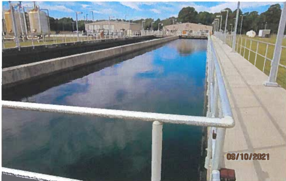
Photograph J - Sedimentation Basins
