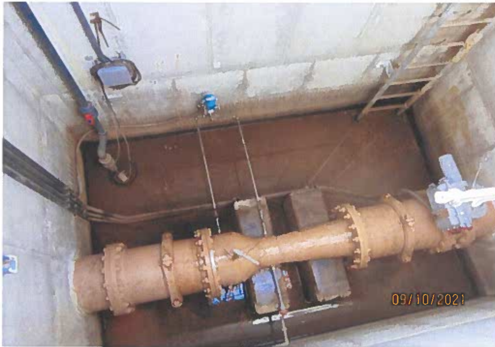
Photograph I - Influent Flow Meter Vault
