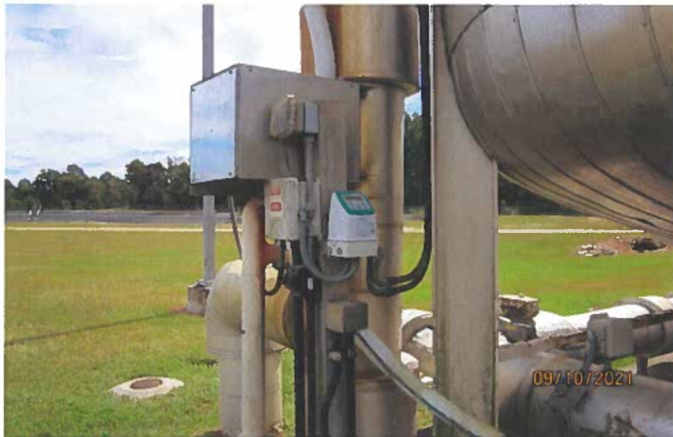
Photograph O – Flow Meters at GAC Filters
