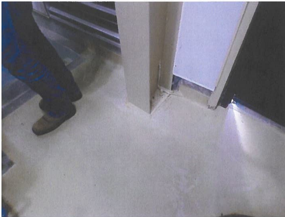
Photograph U - Chemical Building Column Base Plates
