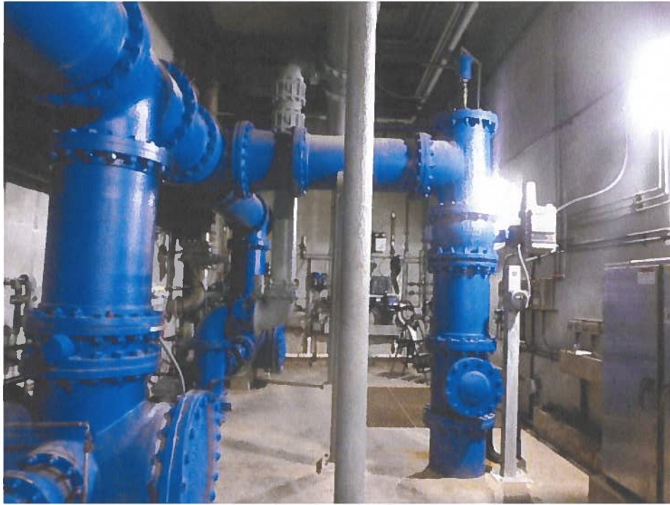
Photograph P – Filter Gallery Walls
