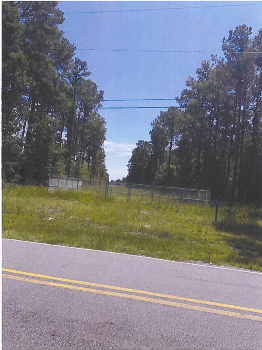
Photograph GG- Interconnect off Blue Banks Loop Road
