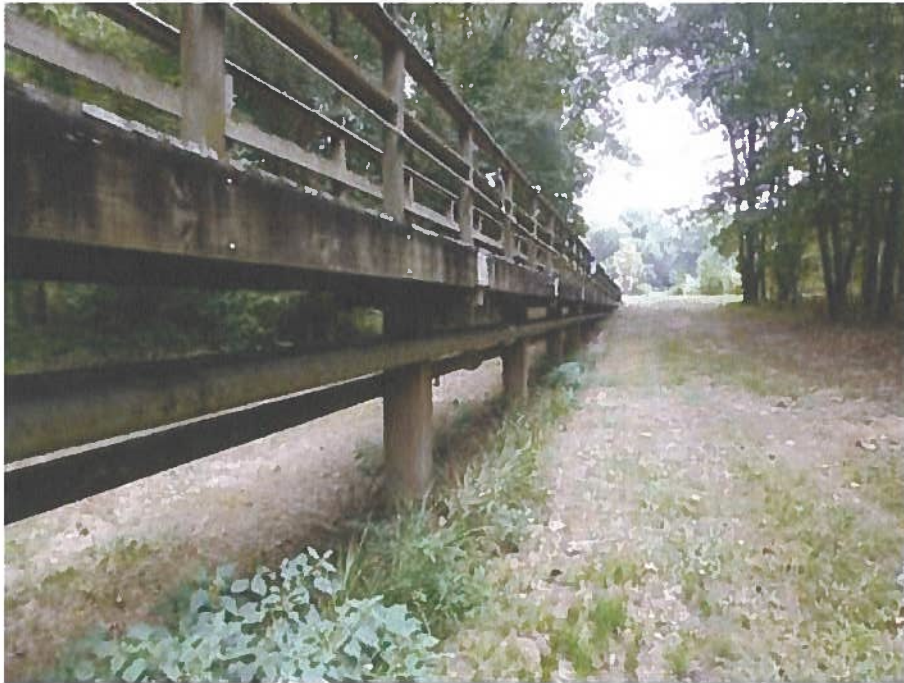
Photograph D – River Access Walkway Underside
