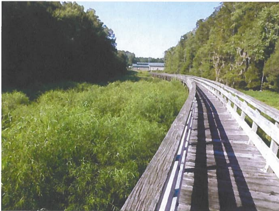
Photograph K- Vegetative Cover Surrounding Pier Prior to Trimming
