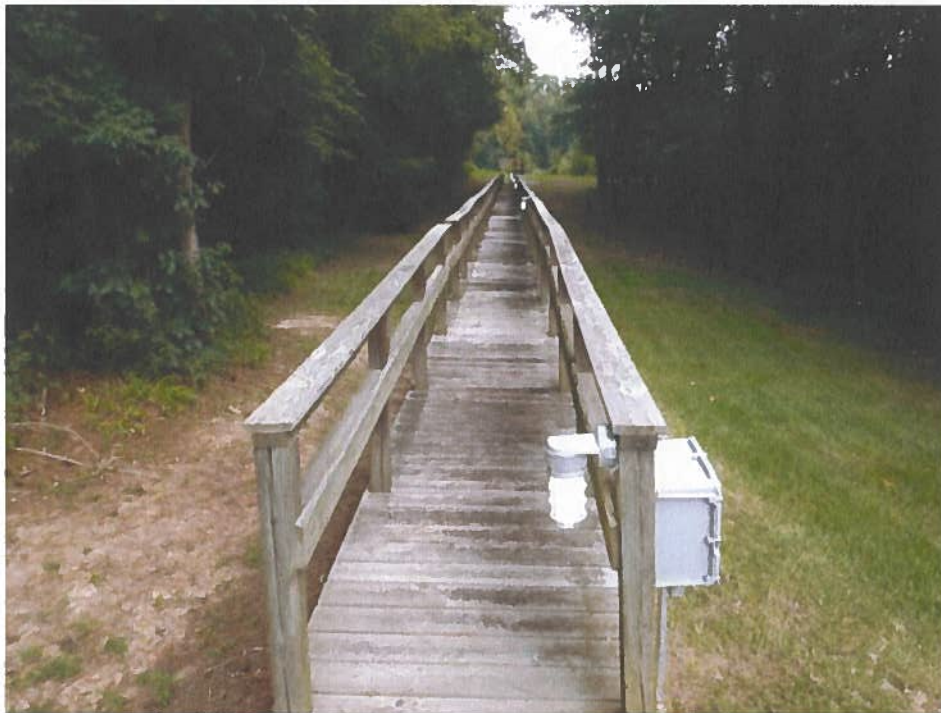
Photograph C – River Access Walkway
