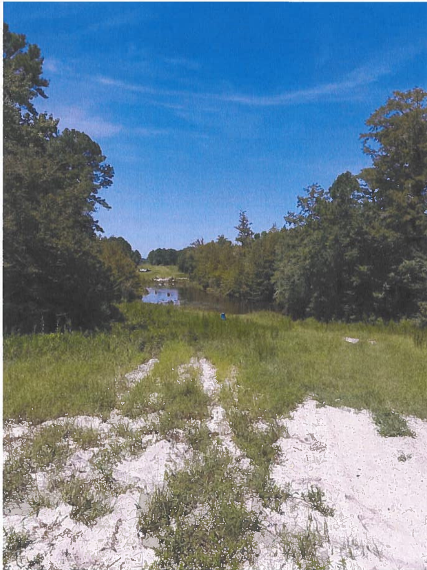
Photograph FF- Old Blow-off on 48" RWM and new Blow-off on 54" RWM
