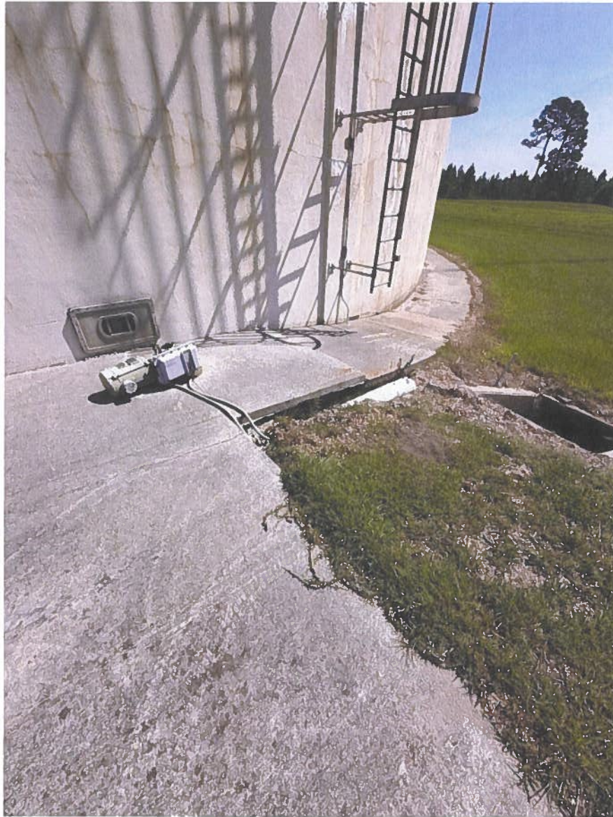
Photograph II- 3 Million Gallon Ground Storage Sidewalk
