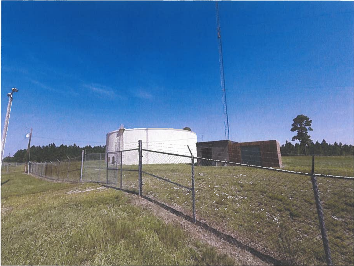
Photograph HH- 3 Million Gallon Ground Storage Tank
