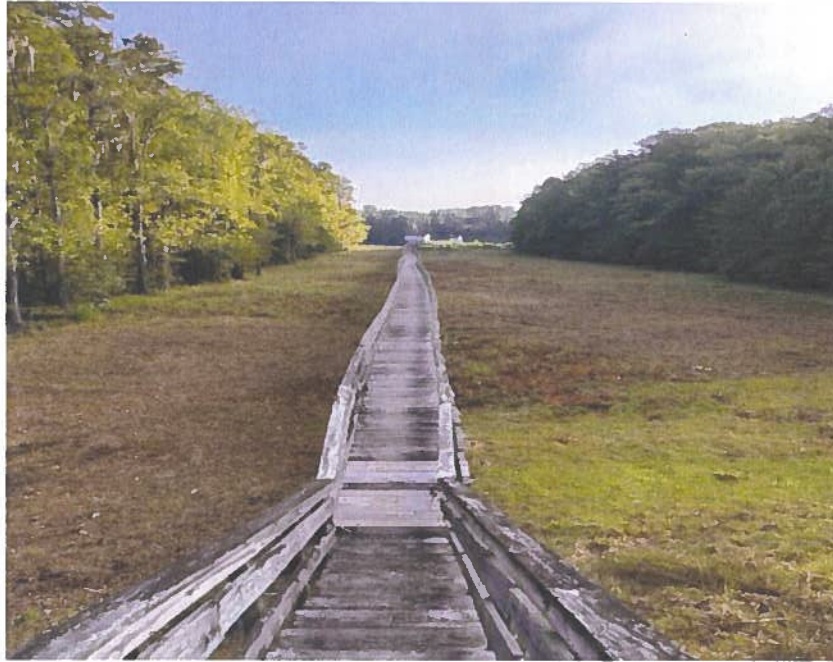
Photograph K'- Vegetative Cover Surrounding Pier Post Trimming
