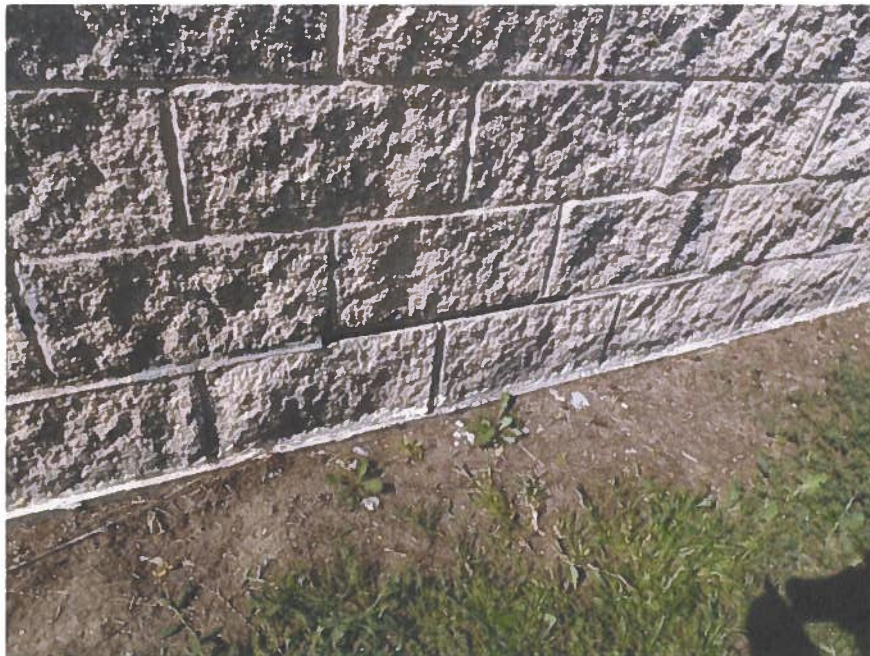
Photograph C –Corroding Masonry Wall Joints
