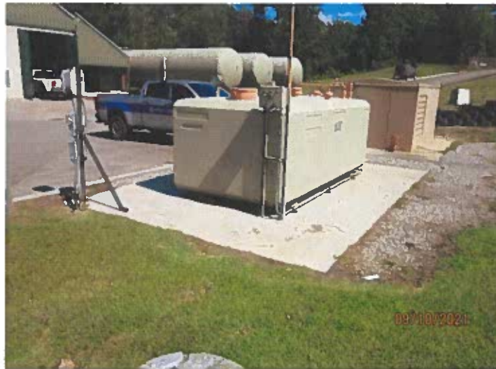
Photograph H - Generator and Storage Tank Require Signage
