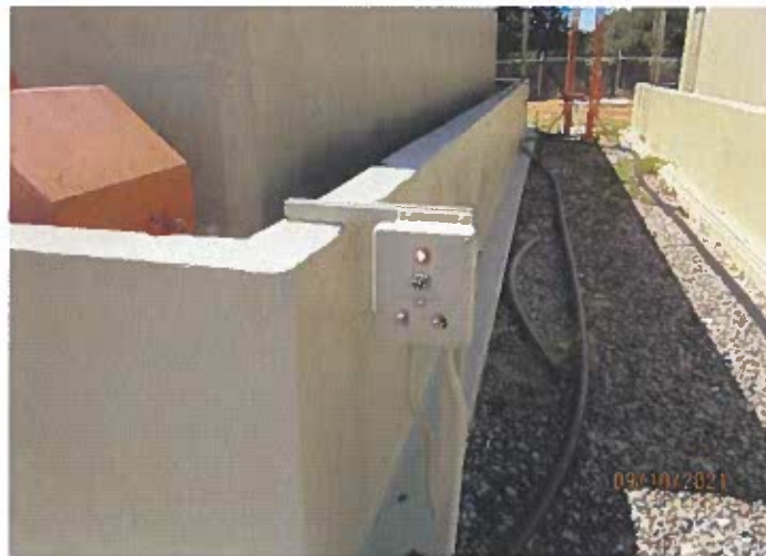
Photograph D – Alarmed Diesel Tank Leak Panel
