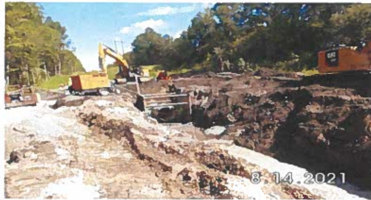
Photograph GG- 54-Inch Steel Raw Water Main Re-Installation in Rattlesnake Branch
