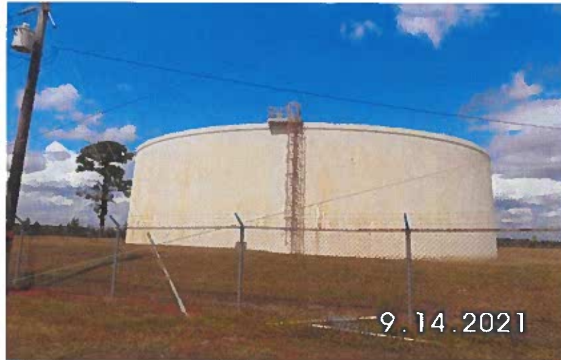
Photograph O – 3 MG Ground Storage Reservoir
