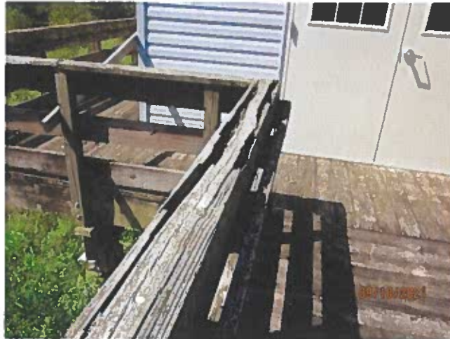
Photograph L- Compromised Dock Handrail
