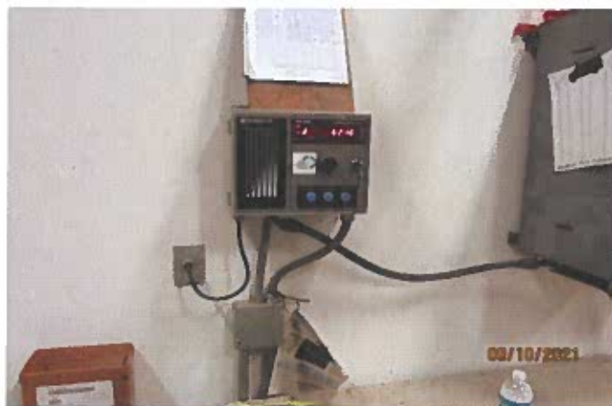
Photograph Q – Pneumercator Panel in Generator Electrical Room
