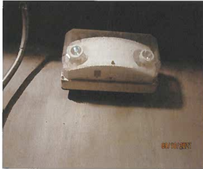
Photograph G – Pipe Gallery Emergency Light Requires Service
